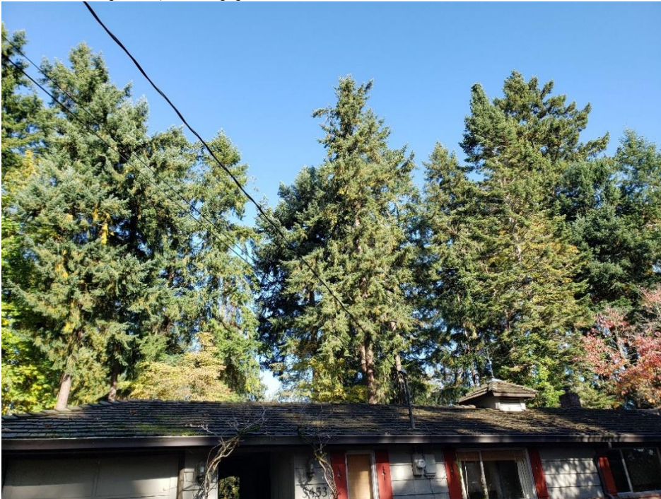
Photo 2. Facing north, showing grove trees located north of the residence.
